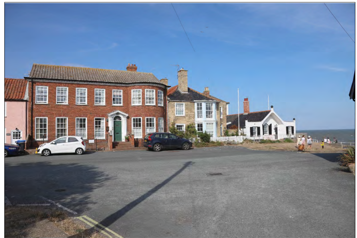
Plate 6) View of Whitehall and Guardship, Southwold (1384422)(right) looking north east
