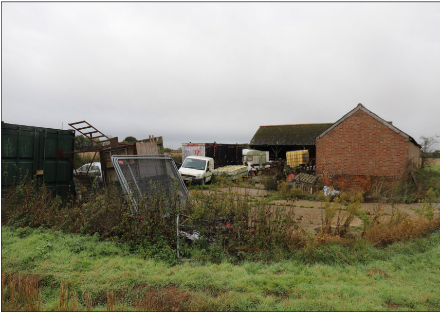
Plate 16) View of the former Mulberry Farm located within SSA East southeast of Little Bromley
