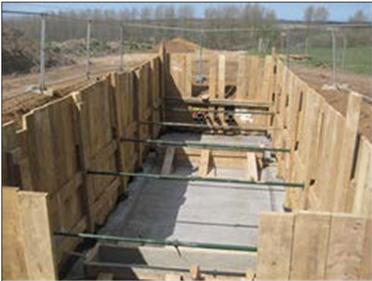
Figure 1.12: A typical jointing pit under construction.
