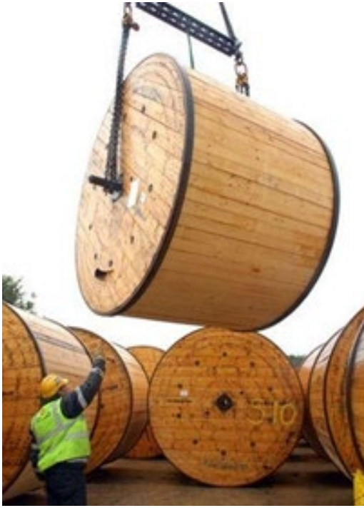
Figure 1.11: Example of a cable drum delivery to cable storage area
