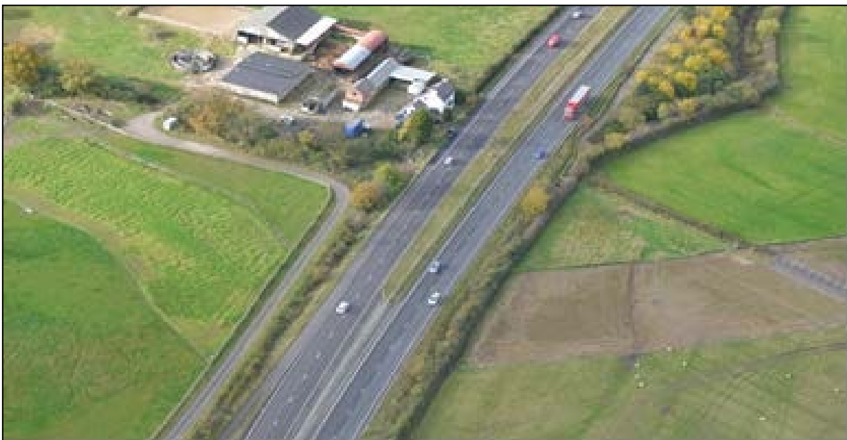
Figure 1.14: Cable corridor during restoration example (RWE renewables UK ltd)
