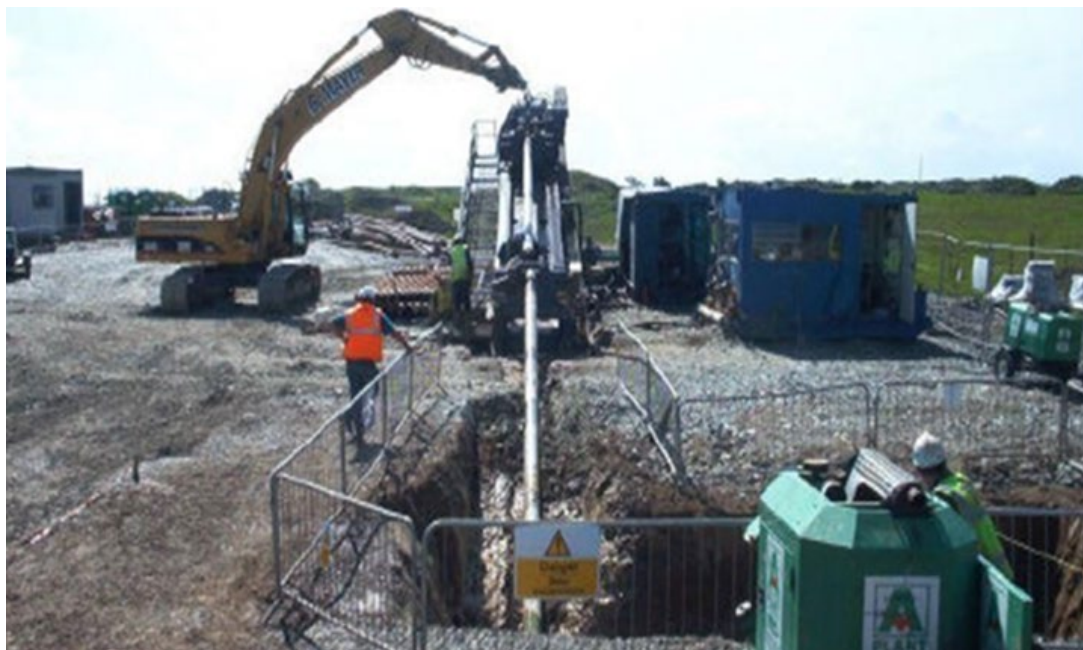
Figure 1.14: Example of typical HDD equipment
