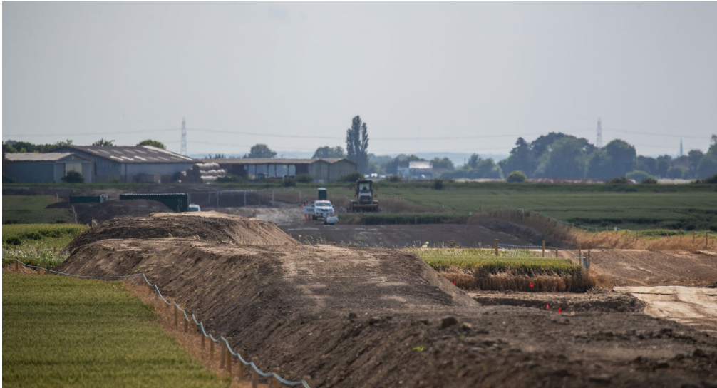
Example of soil storage during construction
