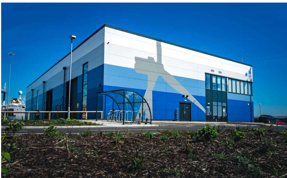
Galloper Operations and Maintenance base
