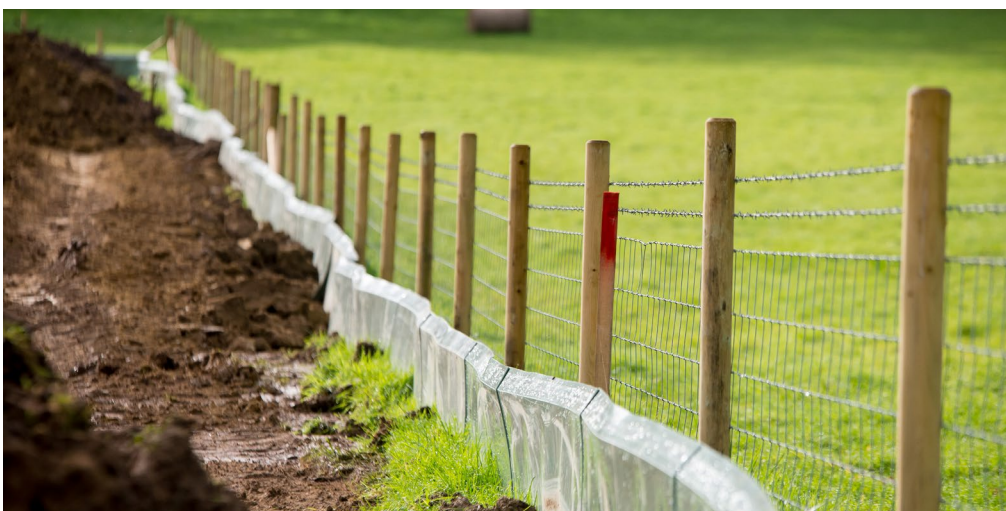
An example of wildlife protection fencing used during construction
