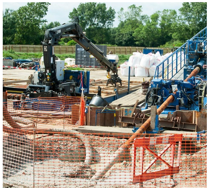
Horizontal directional drilling
