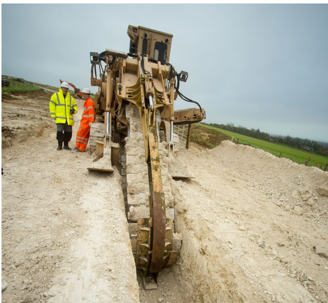
Open cut cable trench excavation
