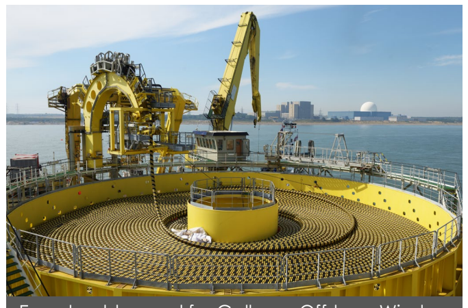
Export cable spool for Galloper Offshore Wind Farm during installation
